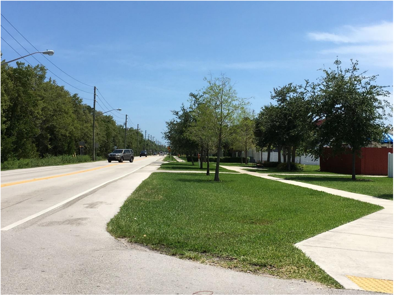
Figure 188. Roadway dry swale
