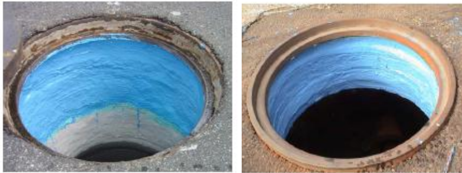
Figure 194. Chimney seal installed (Courtesy USSI)
