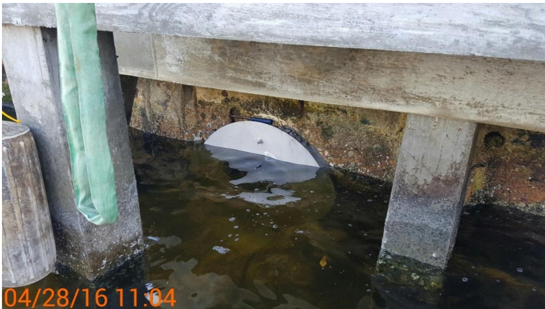
Figure 206. Completed Tideflex installation with insert
