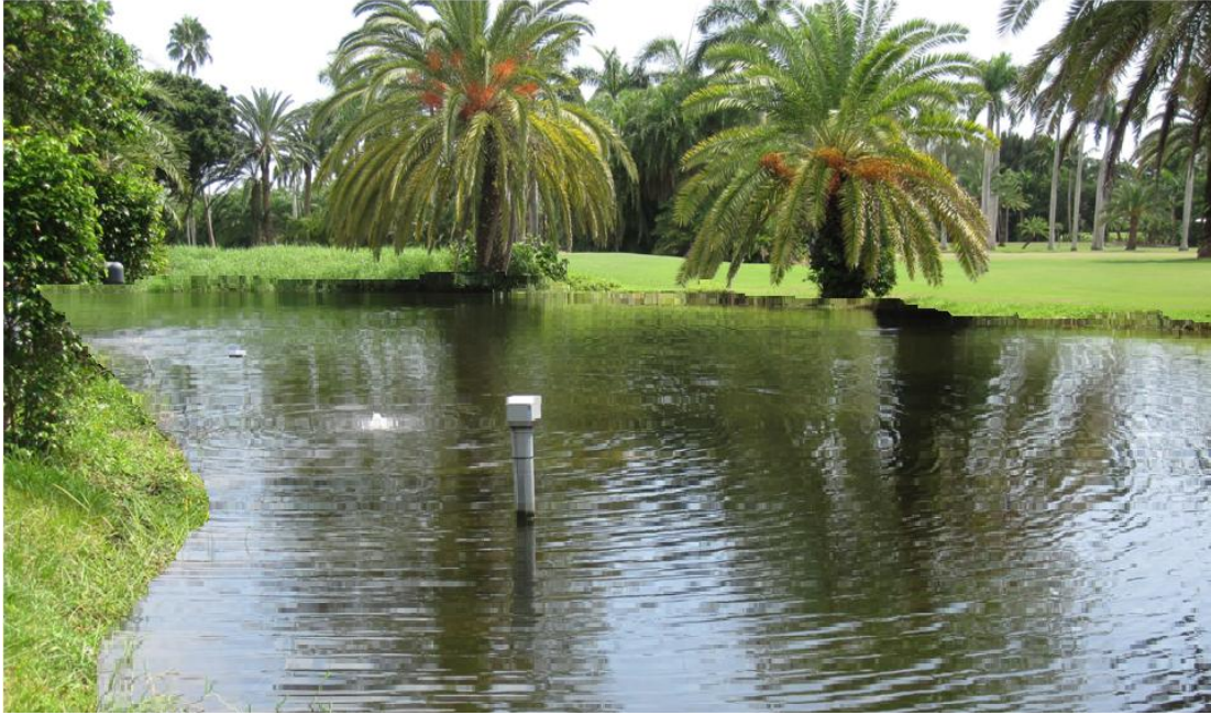
Figure 190. Aerated retention pond
