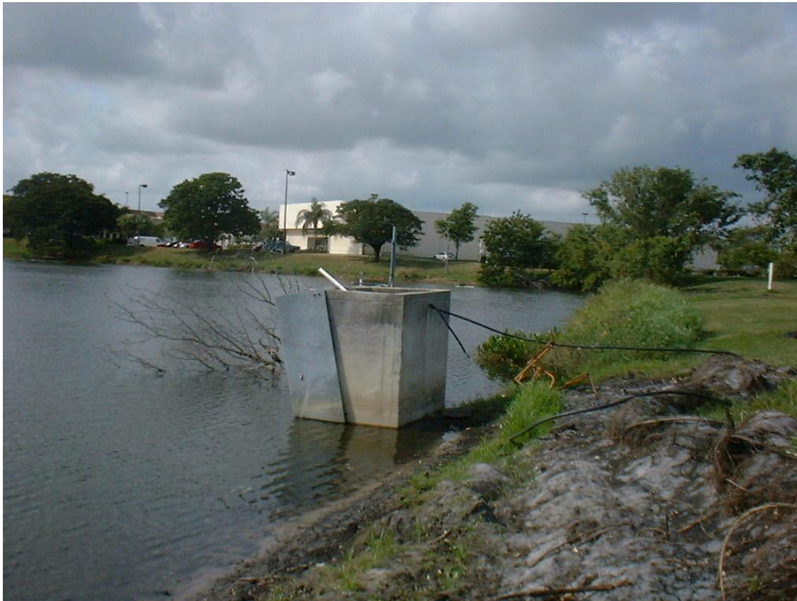
Figure 185. Detention basin with overflow
