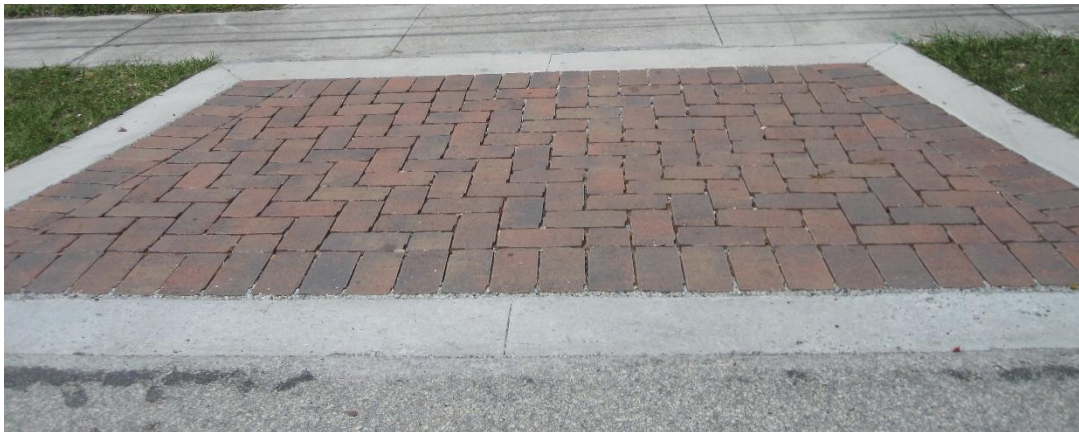
Figure 183. Example of a pervious paver driveway
