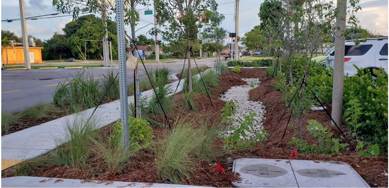
Figure 179. Photo of a bioswale pilot installation in Hallandale Beach, FL ( https://www.hallandalebeachfl.gov/ )
