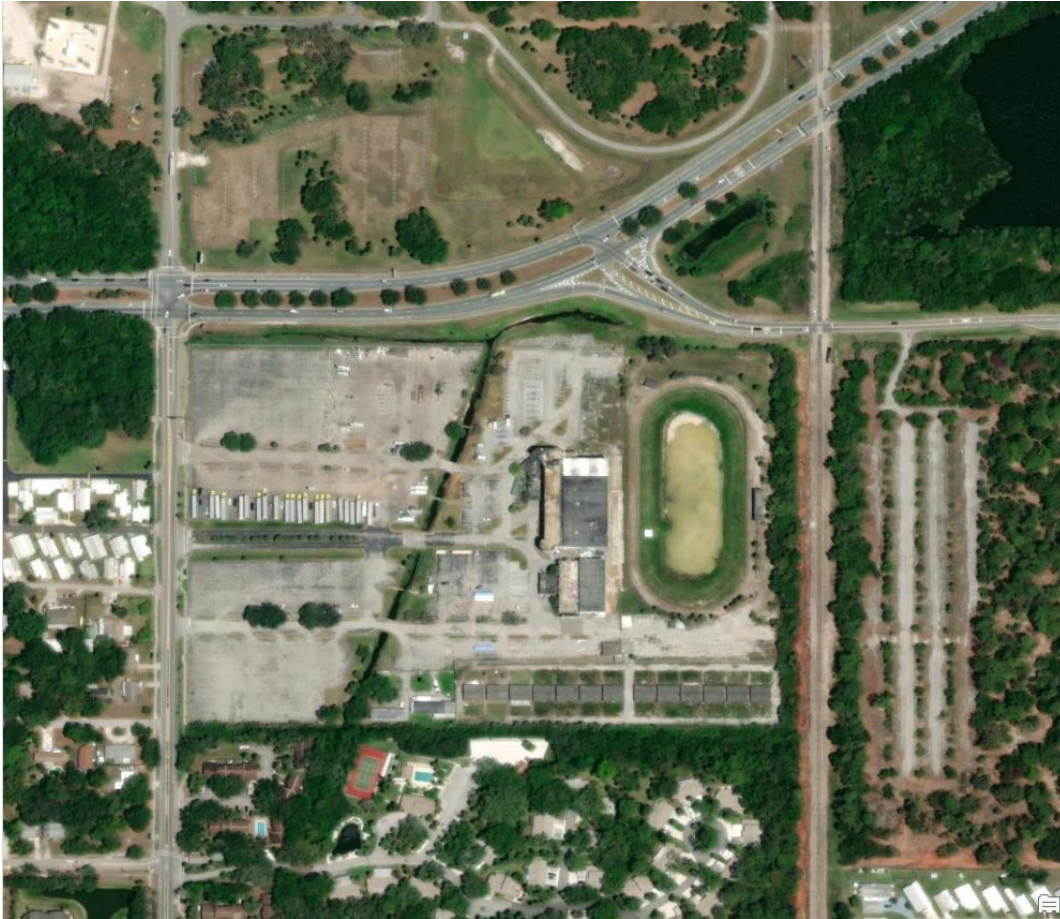
Figure 168. Aerial view of the area north of University Parkway, east of the airport
