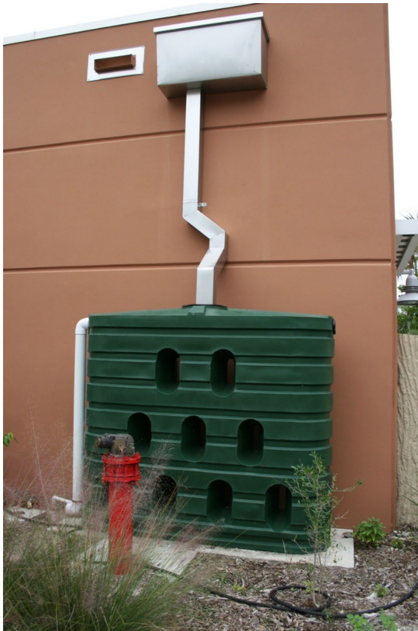
Figure 172. Rainwater harvesting cistern (used for irrigation) at the Pine Jog Environmental Center in West Palm Beach, FL
