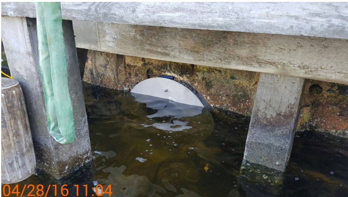
Figure 201. Completed Tideflex installation with insert
