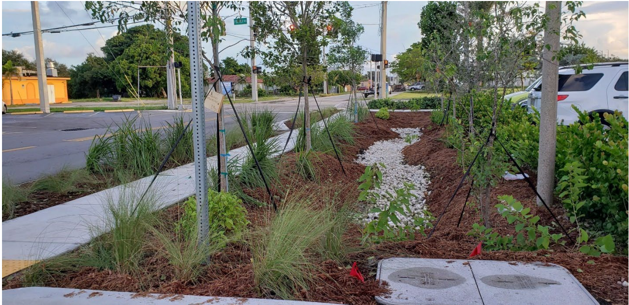
Figure 174. Photo of a bioswale pilot installation in Hallandale Beach, FL ( https://www.hallandalebeachfl.gov/ )
