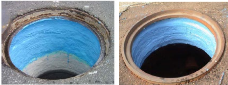
Figure 189. Chimney seal installed (Courtesy USSI)
